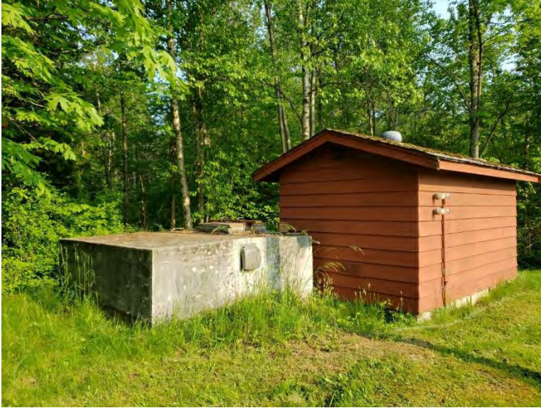
Figure 2: Kelly Rd. Water Assoc. well pump house and adjacent concrete storage tank
